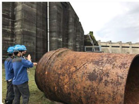
Making an inspection of a water supply station
