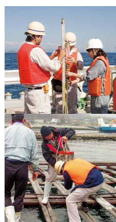
Field investigation for sediment improvement work in the Seto Inland Sea
