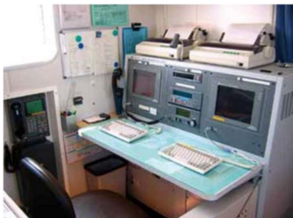
無線区画-1 / Radio equipment area-1
