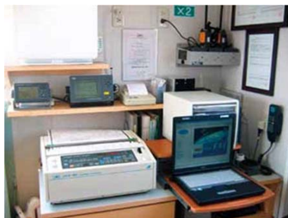
無線区画-2 / Radio equipment area-2
