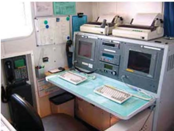
無線区画-1/Radio equipment area-1
