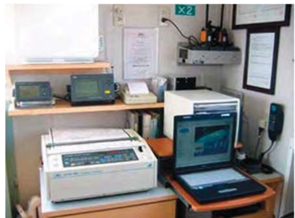
無線区画-2/Radio equipment area-2
