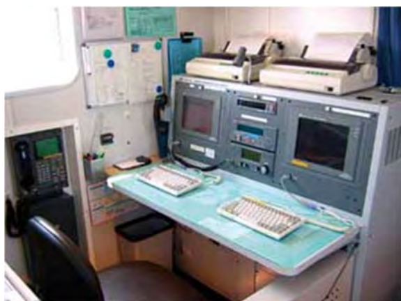
無線区画－1／ Radio equipment area-1
