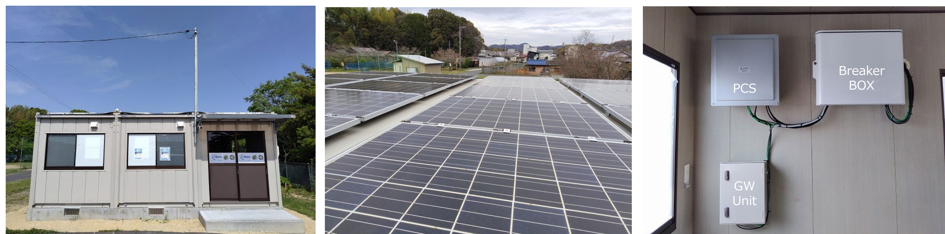
Fig.3 Overview of the facility
