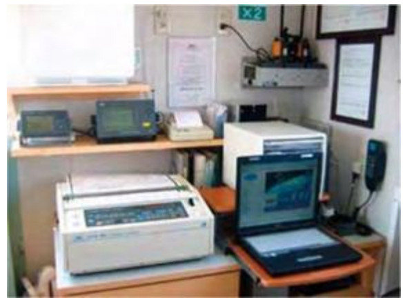
無線区画-2 / Radio equipment area-2
